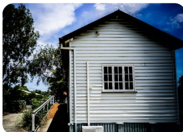
North Ipswich Hub 6 Canning Street North Ipswich
